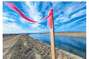
A survey ribbon flutters in the breeze during subsidence repair work in 2021 along the California Aqueduct near Lost Hills in Kern County. (Source: California Department of Water Resources)
