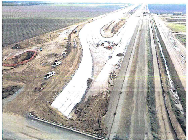
A new section of canal, parallel to the Friant-Kern Canal, had to be built after the canal sank due to excessive groundwater pumping. SOURCE: Friant Water Authority
